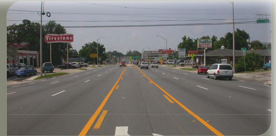
2010 Looking North - Intersection of Pine and 3 rd Street
