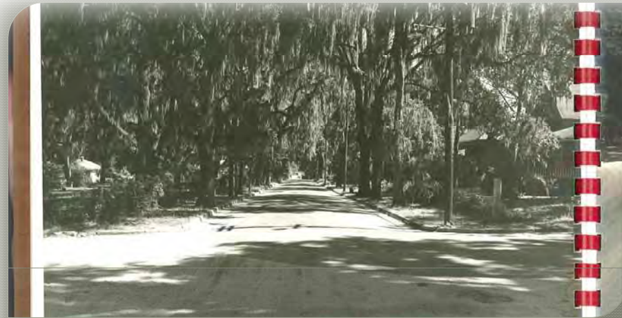
1950 Looking North - Intersection of Pine and 3 rd Street
