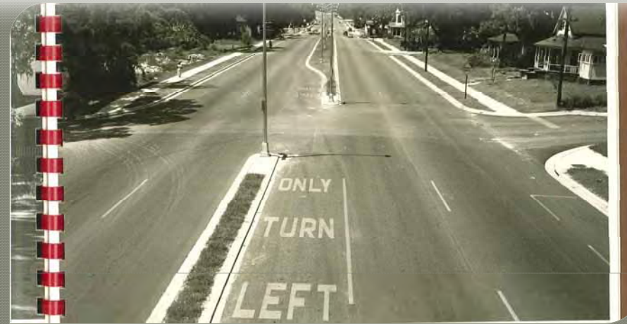
1952 Looking North - Intersection of Pine and 3 rd Street
